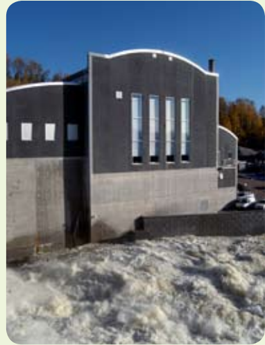
The new Avestaforsen power plant was the biggest investment in hydro power in a decade in Sweden.
