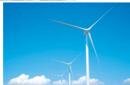
Wind power generation business
