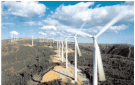
EURUS ENERGY HOLDINGS—THE WORLD'S LEADING DEVELOPER OF WIND POWER GENERATION
