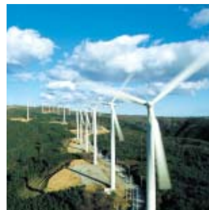
Tomen is steadily laying foundations for expansion of its wind power generation business in Japan and overseas.
