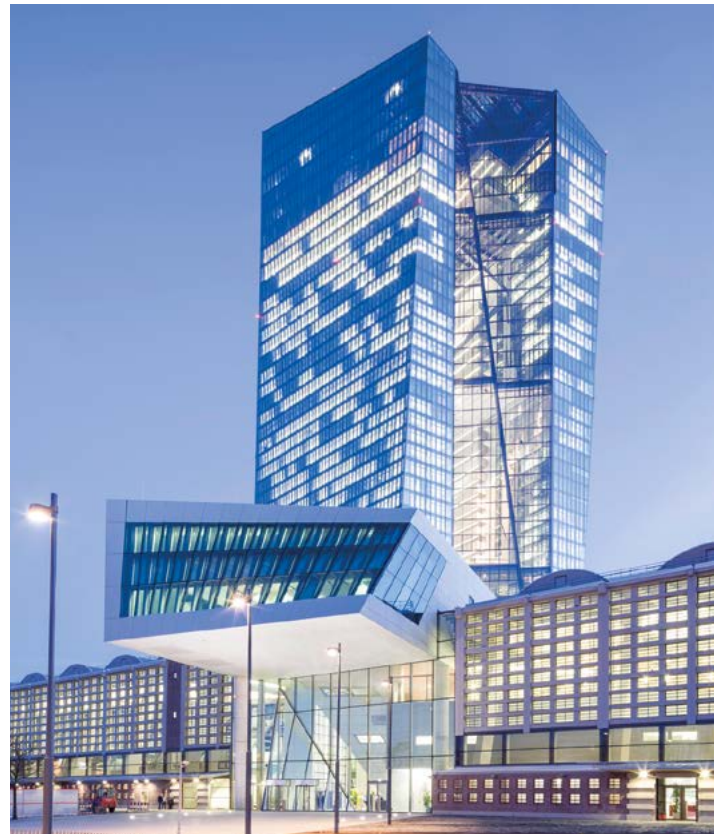
The new European Central Bank headquarters in Frankfurt am Main, Germany, is setting new standards in energy efficiency and sustainability with Uponor's radiant heating and cooling systems.
