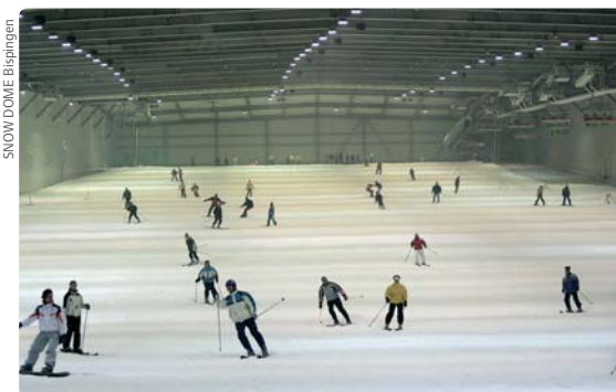
The most modern skiing hall in Europe, Snow Dome in Bispingen, Germany, can accommodate up to 4,600 skiers per hour in the slopes cooled by Uponor solutions.
