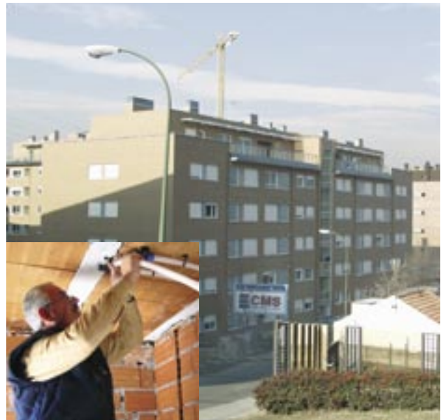
Uponor supplied plumbing systems for 340 homes in a new residential building area near Madrid, Spain, due for completion in the spring of 2005. An engineering firm that decided to opt for Uponor's solution appreciates Uponor's ability to supply a comprehensive package with plastic fittings and the opportunity to make use of installers trained and authorised by Uponor. The system's fast and easy installation gave Uponor a head start over rival systems.
