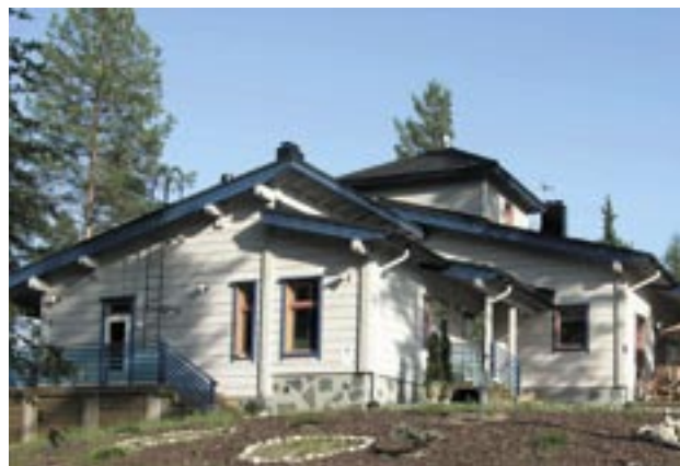
A one-family log house on display in the Finnish Housing Fair was completed on the lake waterfront in the summer of 2004. Concerned with the immediate surroundings and water system, the family opted for Uponor's biological-chemical wastewater treatment plant. The house uses geothermal heating, which distributes heating evenly thanks to radiant underfloor heating. Clean indoor air is guaranteed by a ventilation system, whose hygienic plastic ducts neither absorb dust nor let it circulate in indoor air. The system features a humidity sensor and heat recovery function, which protect the house and save energy. The house serves as a good example of Uponor's wide range of solutions considering that it supplied not only underfloor heating and ventilation systems but also tap water, sewerage and rainwater sewer systems.
