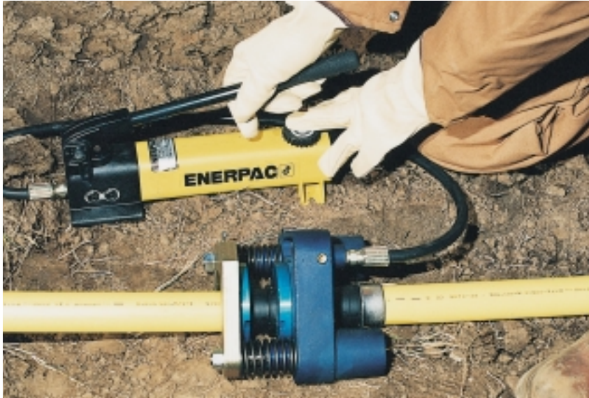
One of the key objectives when developing systems is to make installations more efficient in practice. Uponor provides various joining methods depending on the type of pipe and circumstances of use.
