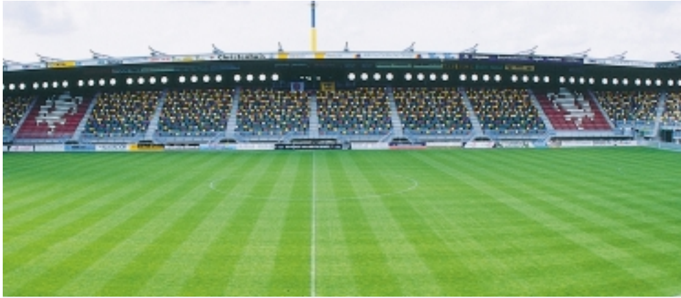
Water-borne heating is increasingly used in outdoor locations such as this football club pitch in the Netherlands. Many of the world's leading sports fields now use Uponor ground heating systems to extend the sporting season and improve playing conditions.
