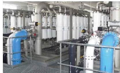
Low pressure RO membrane module for reuse of waste water "HOLLOSEP"
