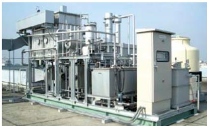
Activated carbon fiber "K-FILTER": Fibrous activated carbon that adsorbs and removes harmful substances and malodorous elements from the air
