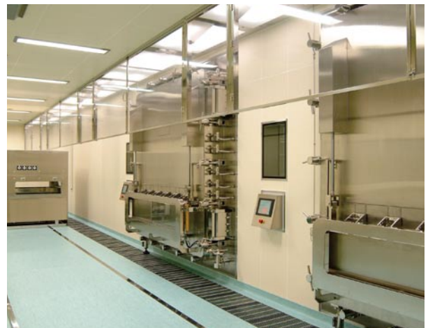
Otsu Pharmaceuticals Plant
