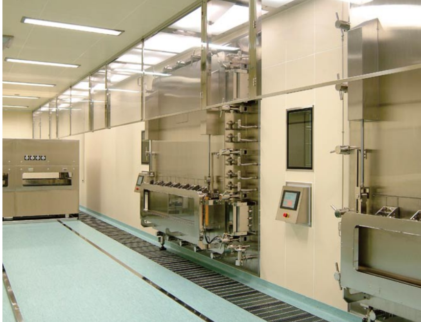
Otsu Pharmaceuticals Plant
