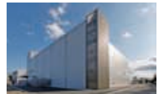
A Pharmaceutical Raw Material Building
