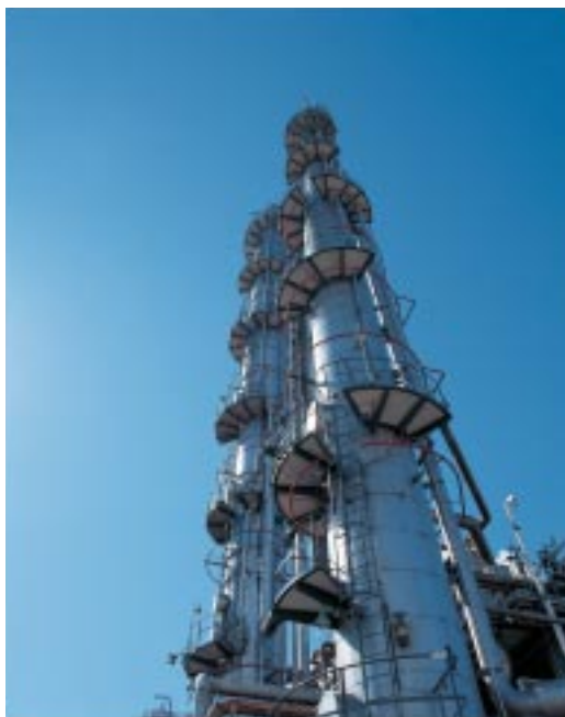
Distillation tower at Kyowa Yuka's Yokkaichi Plant
