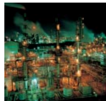
Kyowa Yuka's Yokkaichi Plant
