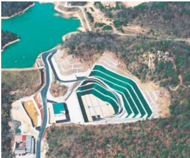
Landfill liner for waste-disposal sites
