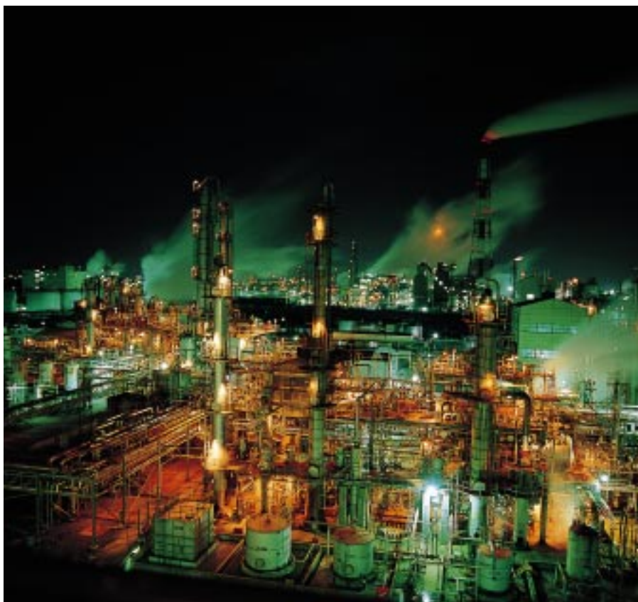
Kyowa Yuka's Yokkaichi Plant
