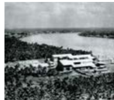
A factory at the time of Ajinomoto Co. (Thailand), Ltd.'s founding
