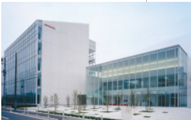
Food Products Global R&D Center (Photo from Kokyu Miwa Architectural Photograph Laboratory)
