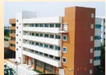
Thai Technology and Engineering Center
