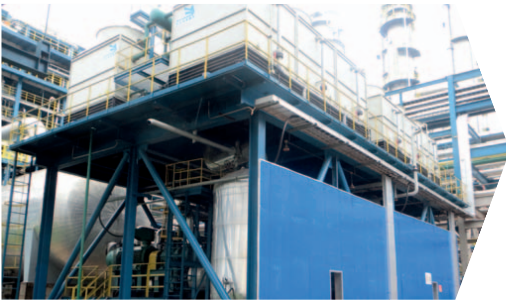
The above picture shows the low-temperature thermal-energy power generation by hot water at Sinopec Hainan Refinery Co., Ltd.,
