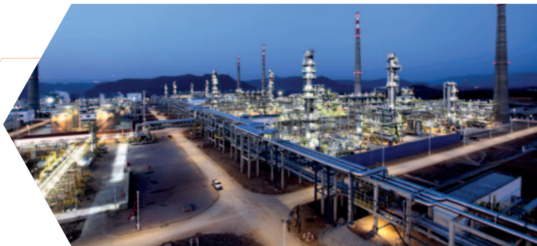
The above picture shows the Sinopec Yuanba Natural Gas Process Plant Project
