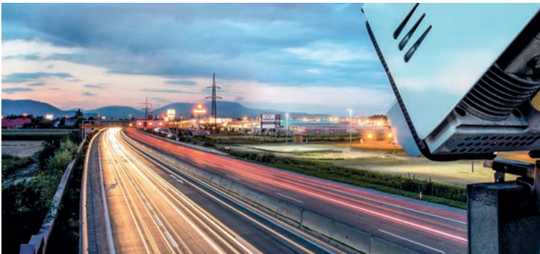
Fully automatic control systems function without interrupting the traffic flow.
