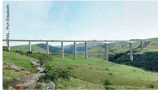
Bridge over the river Mtentu – after completion, it will be Africa's highest bridge.
