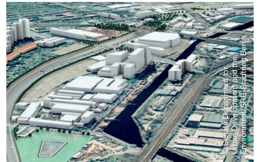
View: Panel 5 from the north
