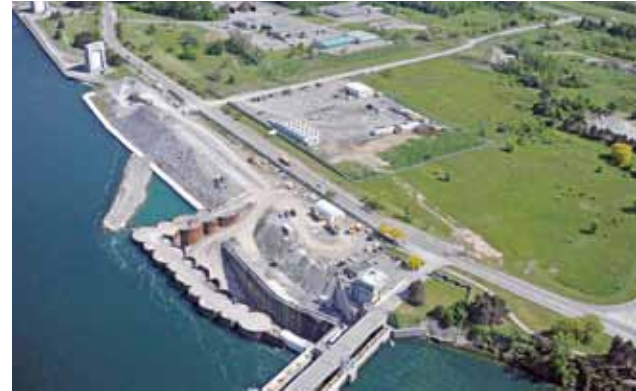
Construction of Niagara Tunnel Project
