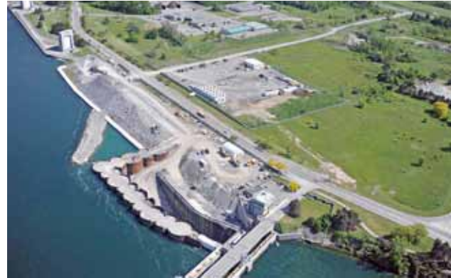
Construction of Niagara Tunnel Project
