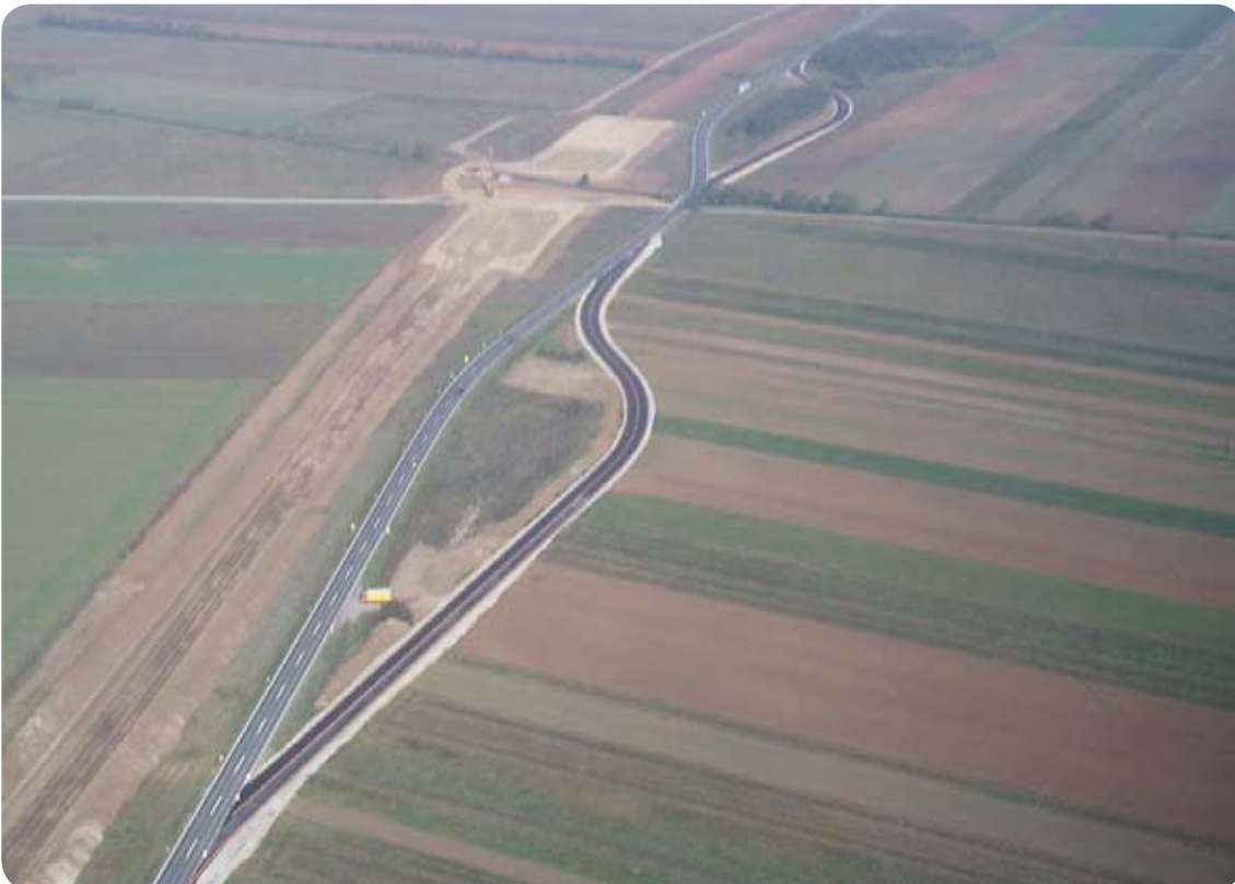
Northeast-motorway A6, Bruckneudorf-Kittsee, Austria
