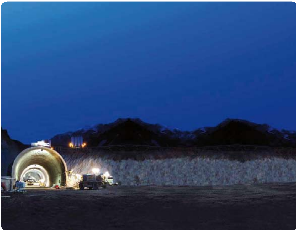
Railway Tunnel Brixlegg, Austria
