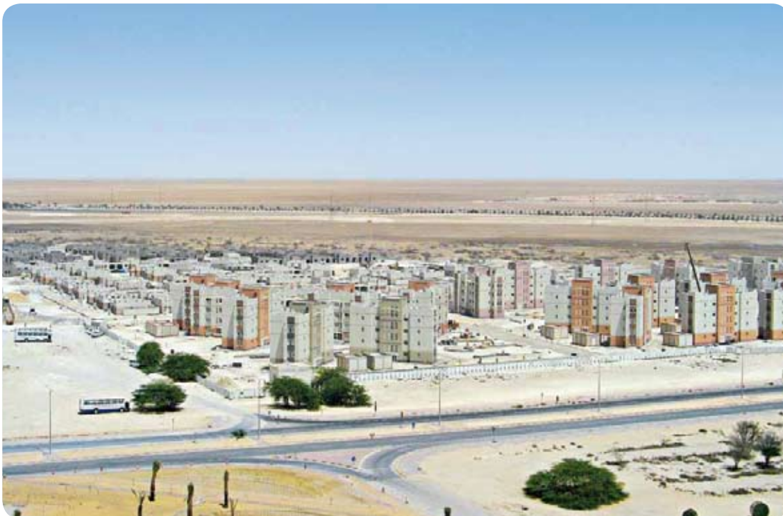
Mesaieed Housing Project, Mesaieed, Qatar
