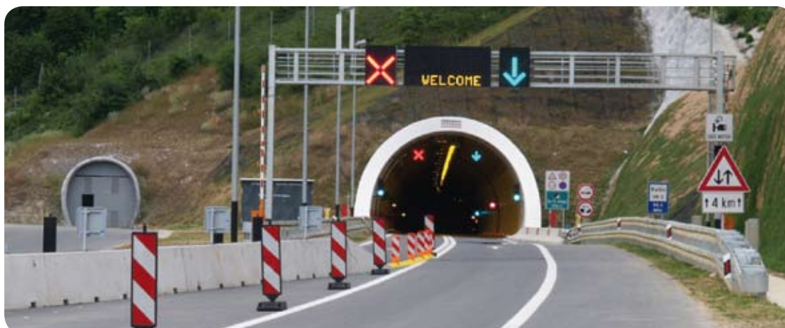
Motorway Zagreb-Macelj, Tunnel Tri Kralja, Croatia
