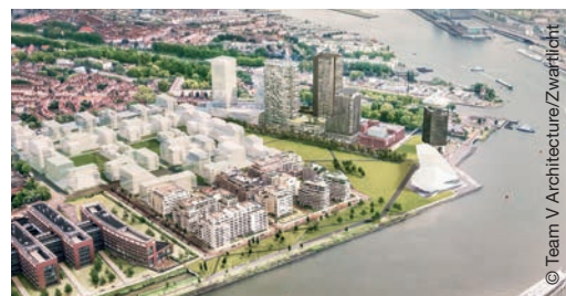
STRABAG subsidiary ZÜBLIN to build the large-scale project Congresshotel & Residential Tower Overhoeks in Amsterdam.
