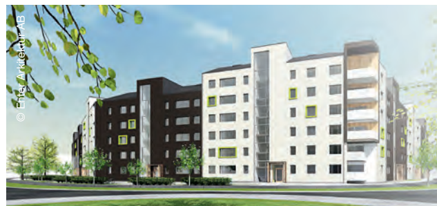
NIMAB project "Alvine" in Malmö (Sweden)
