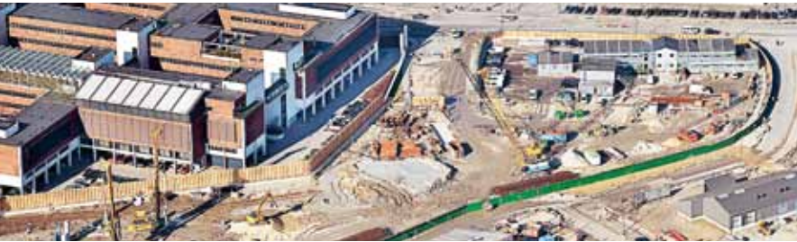
Construction of a 2 km metro tunnel
