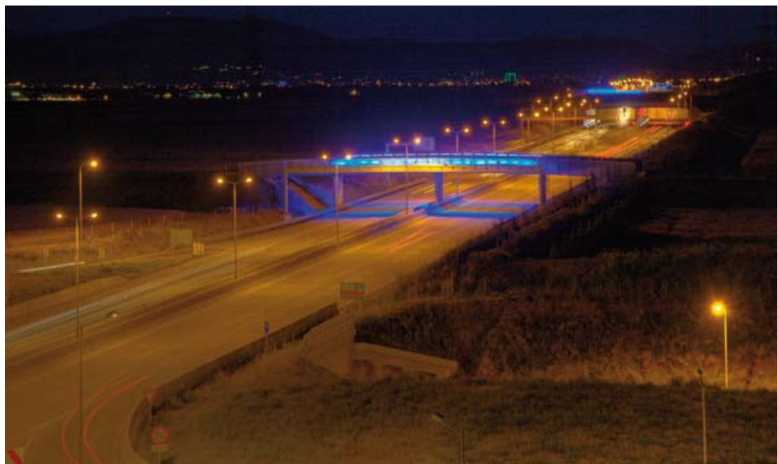
EXPRESSWAY S1, SCHWECHAT/RANNERSDORF, AUSTRIA
