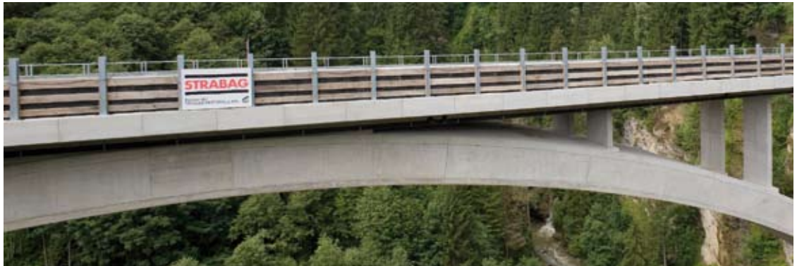
ANGER GORGE BRIDGE, BAD HOFGASTEIN, AUSTRIA
