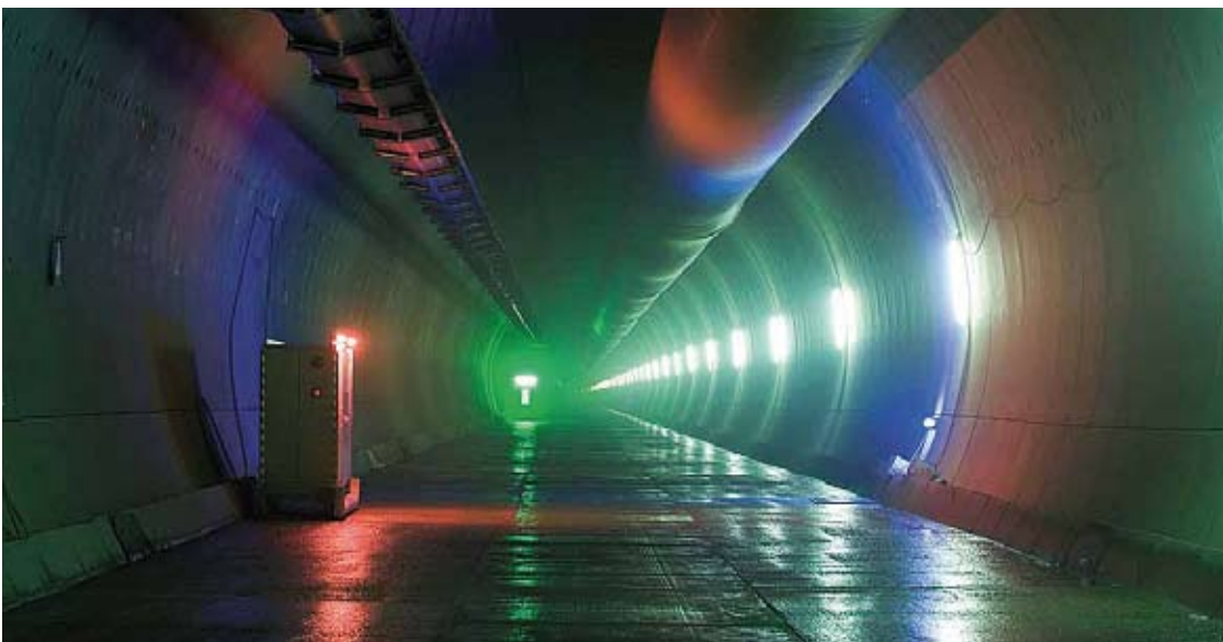
ISLISBERGTUNNEL, UETLIBERG WESTERN KNONAU, SWITZERLAND
