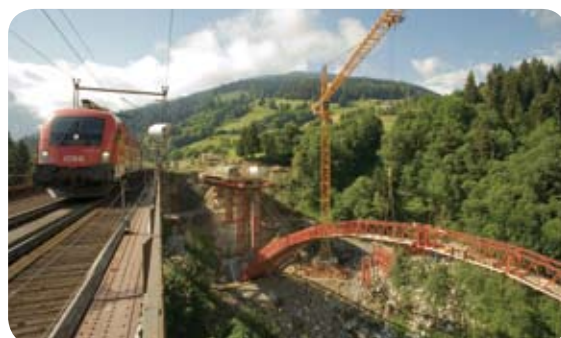
Railway bridge, Angerschluftbrücke, Bad Hofgastein, Austria
