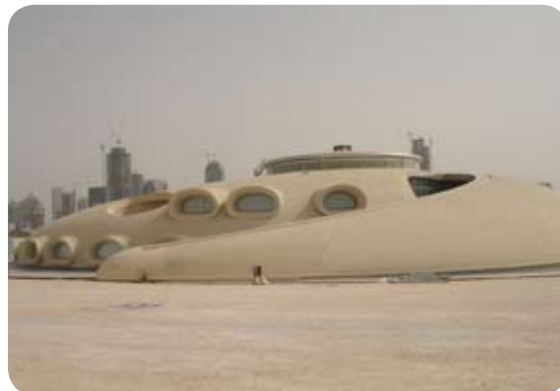
Private Beach Villa Project, Qatar
